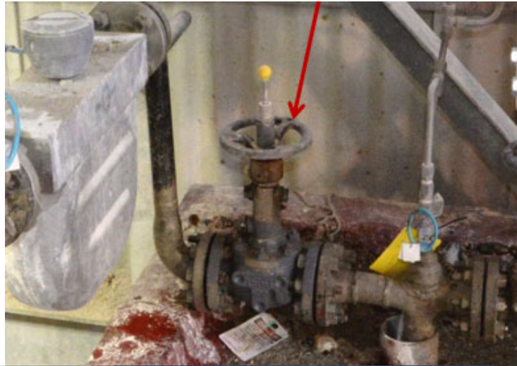
ORBIT® Valve on Ammonia Feed to Granulator
